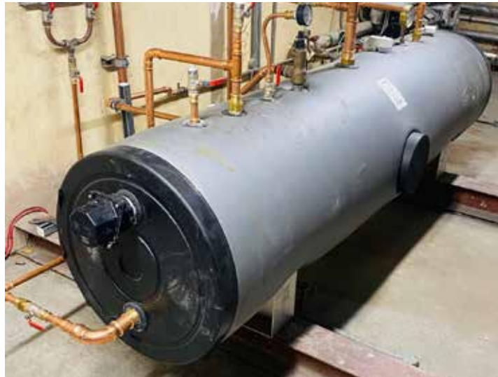
Buffer vessels for hot or chilled water with standard sizes up to 5000 litres
