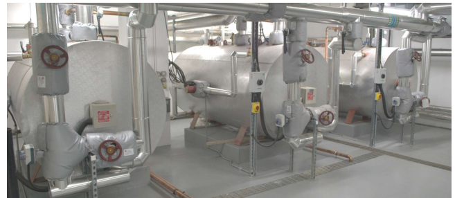
Above: Rycroft Storage Calorifiers at the Mater Hospital, Dublin.
