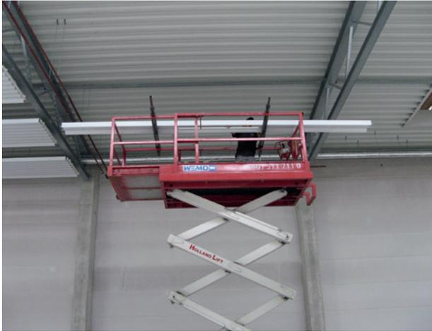
Figure 6. Panel resting on foam on scissor lift
