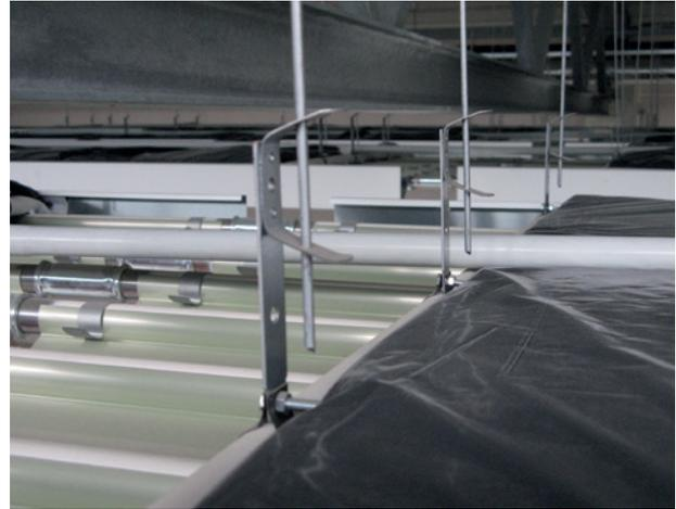
Figure 7. Spring fixing hanging brackets fitted
