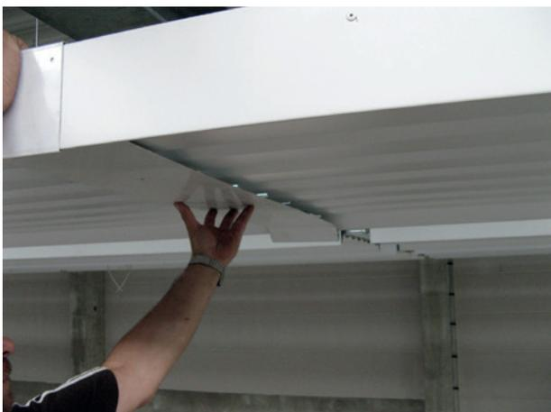
Figure 9. Centre coverplate being fixed
