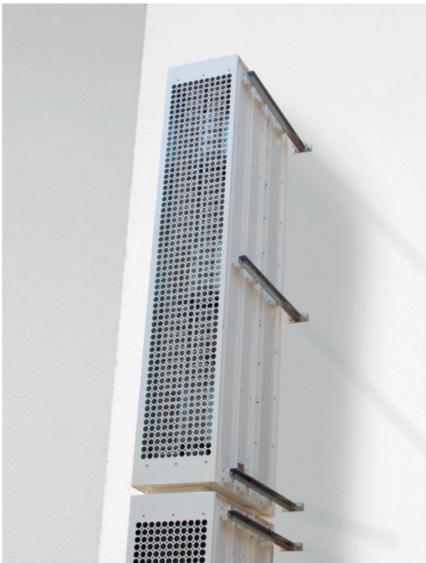
Vertically mounted stacked units via Unistruts and Vertical Mounting Plate
